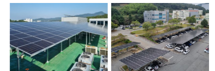
Solar Power Plant Installation in Daedeok DC
